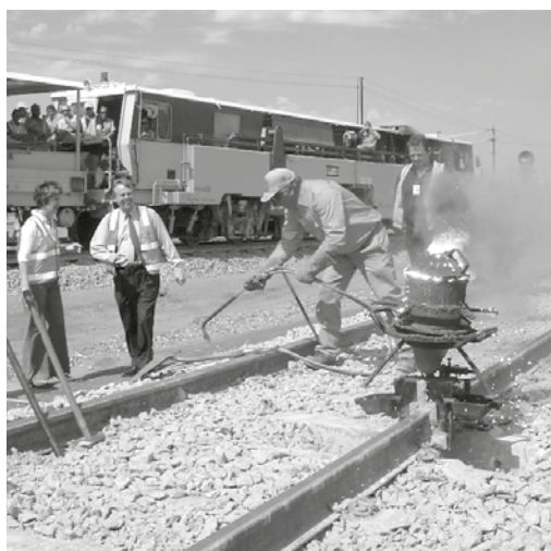
Figure 1 Molten iron is formed from aluminium and iron(III) oxide.
